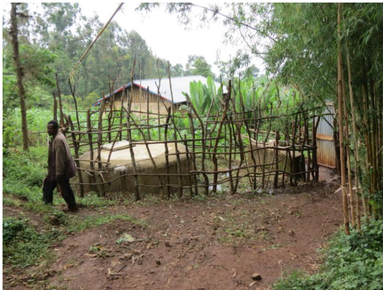
Ele gravity scheme collection tank and first water point.
