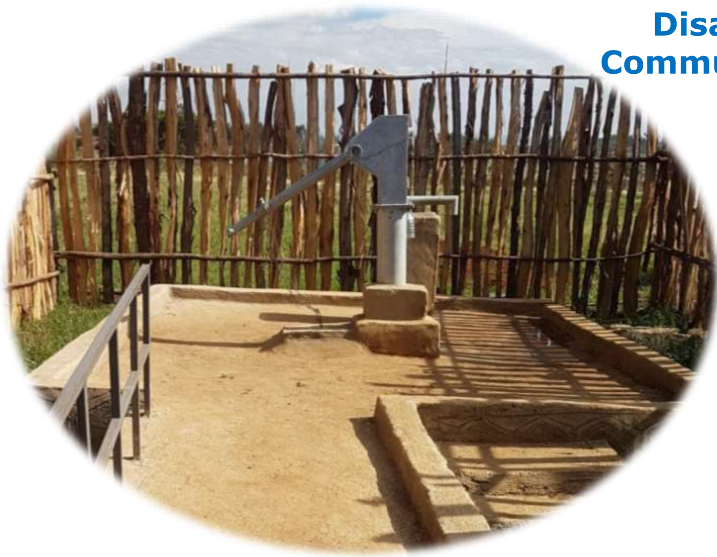
Hand dug well fitted with hand pump
