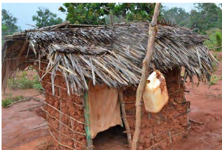
Local Latrine with HWF, Kilifi, Kenya
