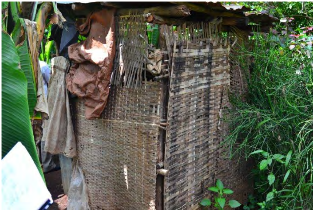
Local Latrine, Shebedino, Ethiopia
