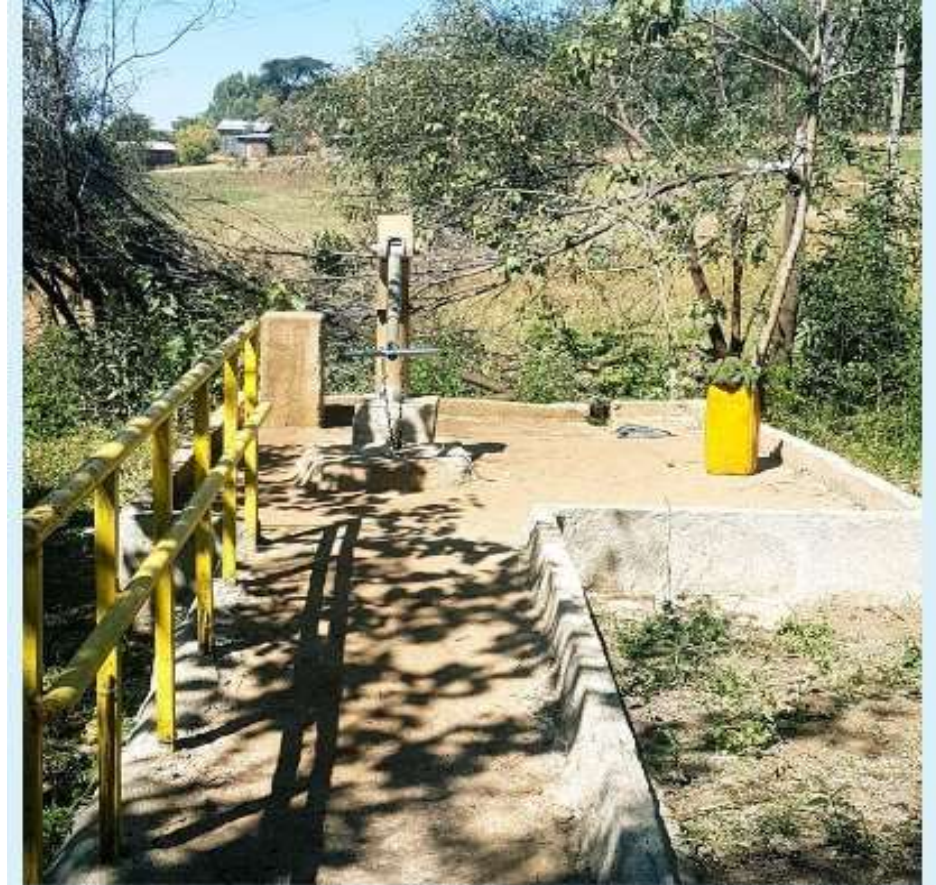
Rehabilitated and accessible hand dug well in Bahir Dar Zuria woreda, Amhara region.
