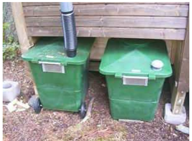
Figure 15. Movable ventilated collecting bins with overflow for leachate discharge (source : PikkuVihreä, Finland)
