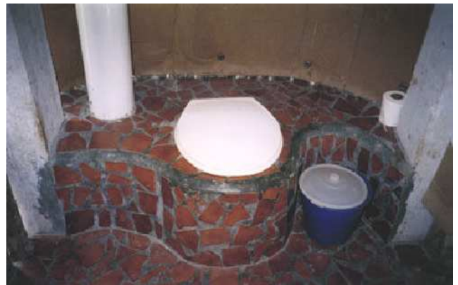
Figure 8. Owner-built toilet seat with storage for wood chips to cover the pile on a daily basis (Puerto Morelos, Mexico) (source: The ReSource Institute, see below).
