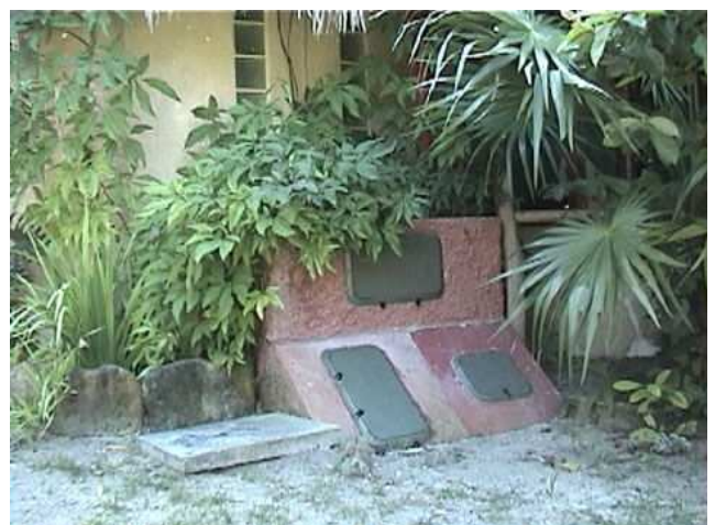
Figure 9. Owner-built single-vault composting toilet with built-in toilet connection and outside access for maintenance and discharge (Puerto Morelos, Mexico) (source: The ReSource Institute, see below).
