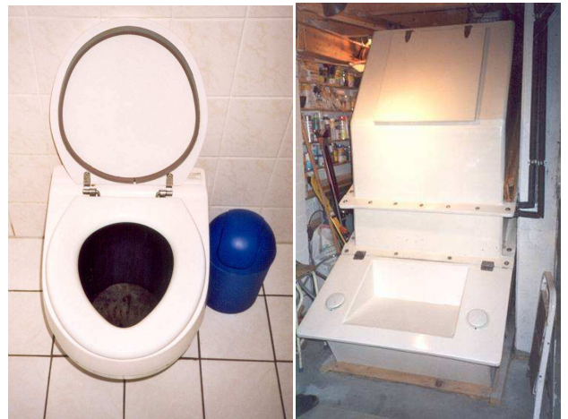
Figure 7. Left : Dry toilet with removable insert and sealed toilet seat. Right : Insulated single-vault composting container with upper lid for maintenance and lower lid for discharge and working platform (both Hamburg-Allermöhe, Germany, source: Berger and Lorenz-Ladener, 2008).
