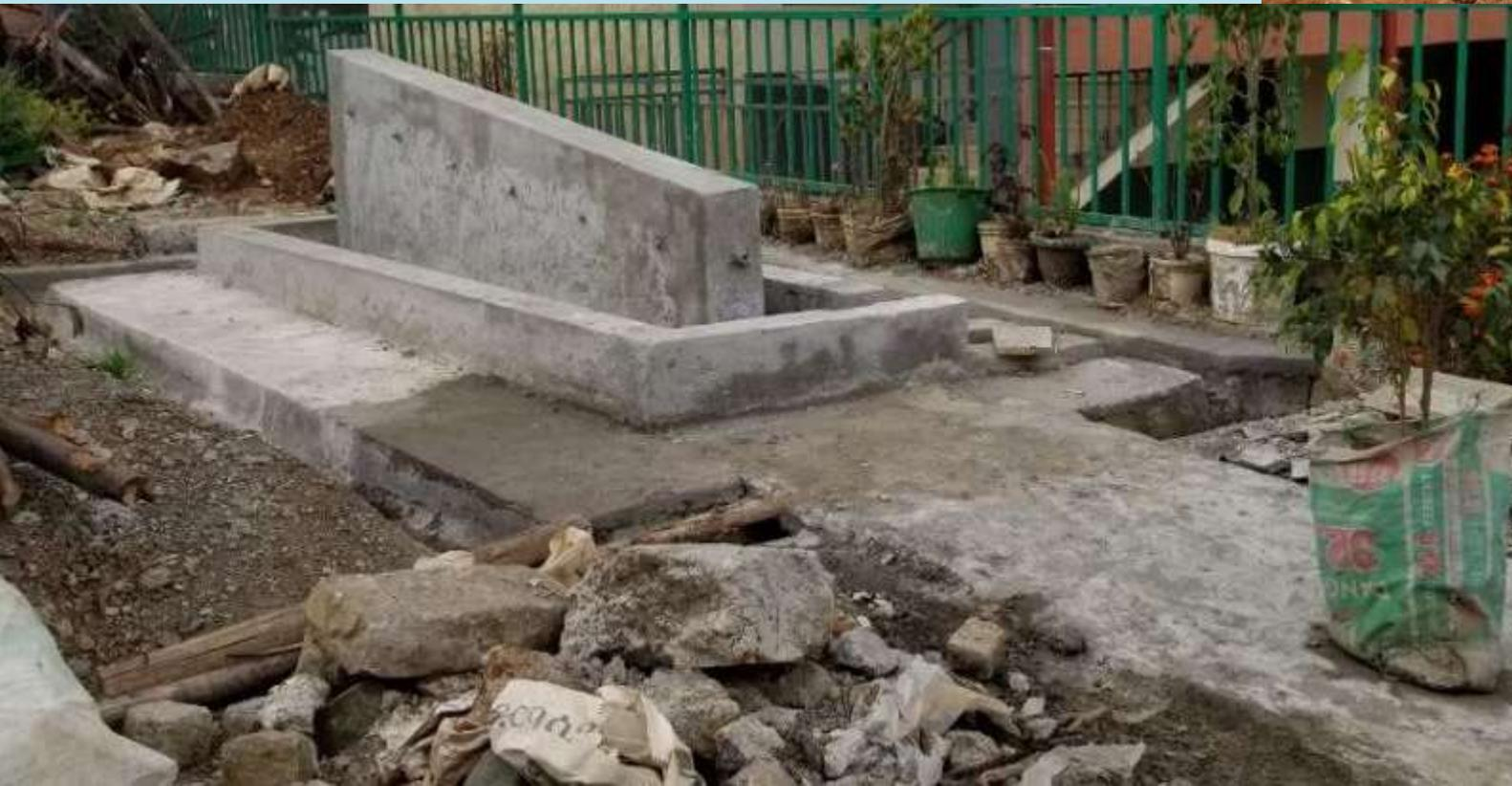
The ramp should be placed in front of the (lower) tap, meant for the child with disabilities.
