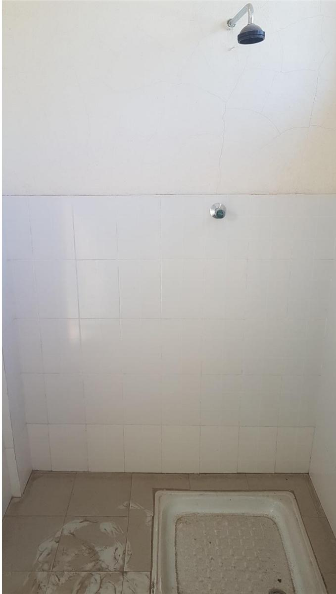
The shower/MHM room in the girls latrine needs to be also made accessible. The floor does not have a step like the WaterAid construction, but lacks a seat, handrails and a lower tap.
