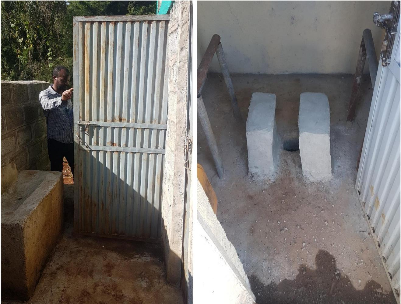
When the door opens to the inside once you have entered the room with the wheelchair, it is impossible to close it (as seen on the right above). Therefore, the door has to open to the outside.
