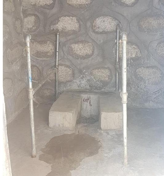
For a person using a wheelchair and many others with physical disabilities having handrails next to the seat on both sides is necessary in order to transfer themselves on the raised seat from the wheelchair. Without the handrails it can be impossible or very difficult for them.
