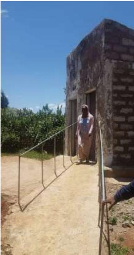
The second one (Murango Geso) had a nice ramp and entrance, but because the ramp was constructed diagonally to the facility, the entrance was too narrow.
