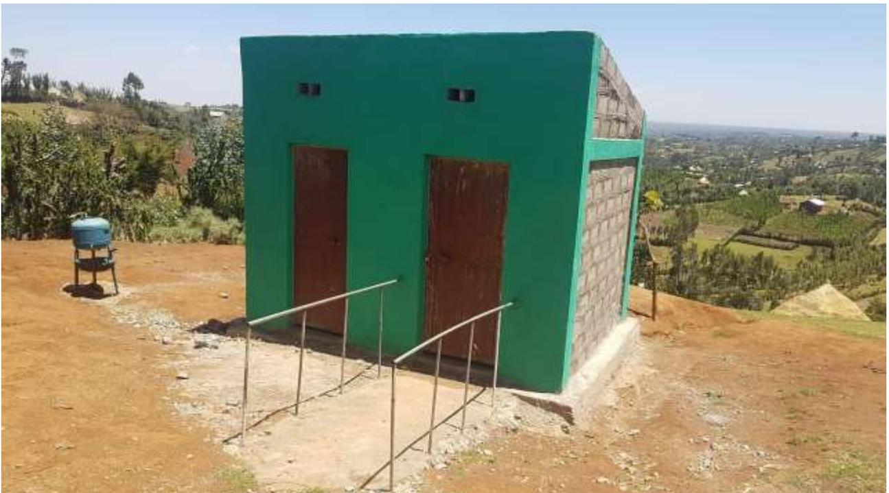
The first (Harbegata) one had a nice ramp and raindrails leading to the facility, but a step remained just at the entrance. Inside the facility the raised seat and handrails were not there. The CMP supervisor and health focal person were aware of the problem and promised to fix these and also to add a path to the facility from the health post before the final payment.
