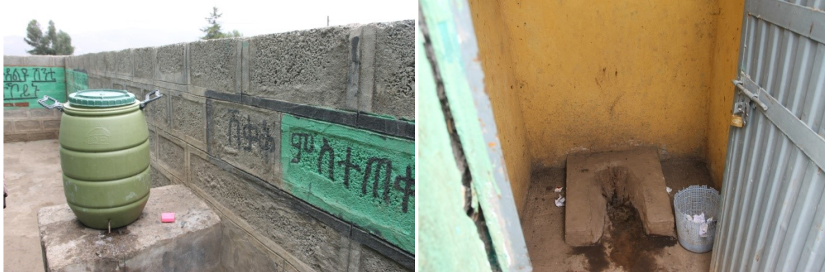
Figure 6: Sanitation Facilities for Girls
