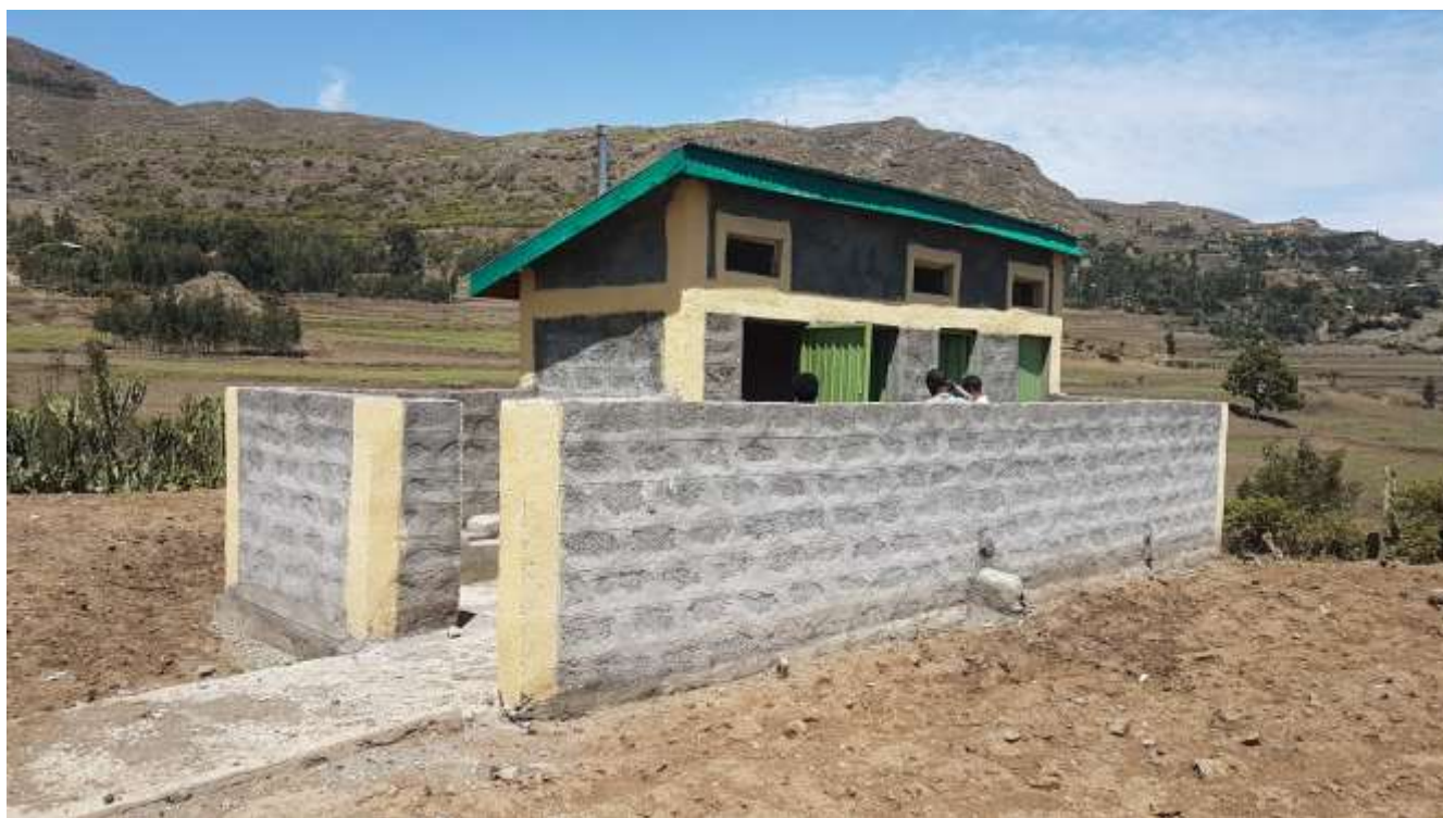
Jonamora elementary school latrine in Endamehoni woreda
