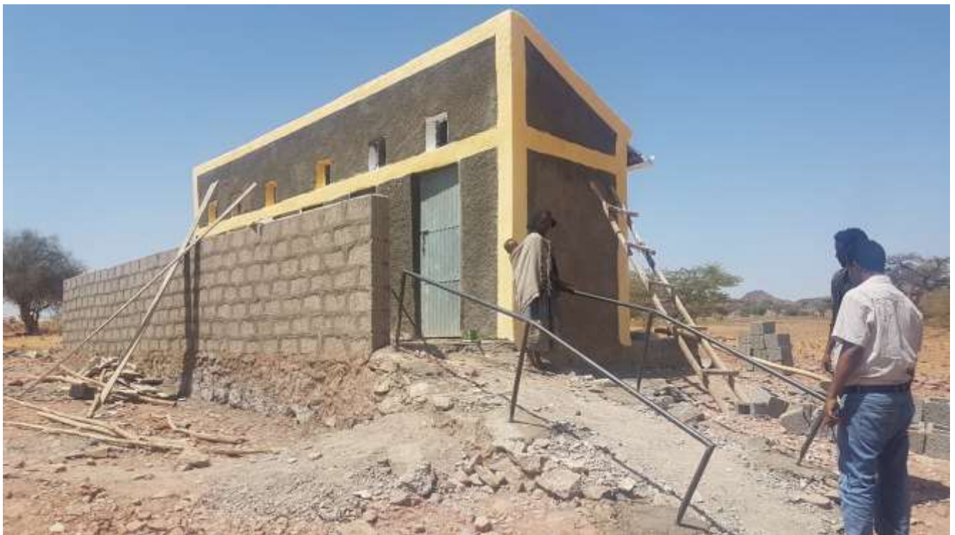
Assessing the school toilet ramp under construction in Seharti Samre woreda
