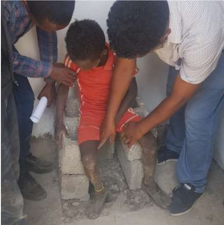
The CMP supervisor and RSU team leader practically testing the toilet seat and adjusting it to fit children better
