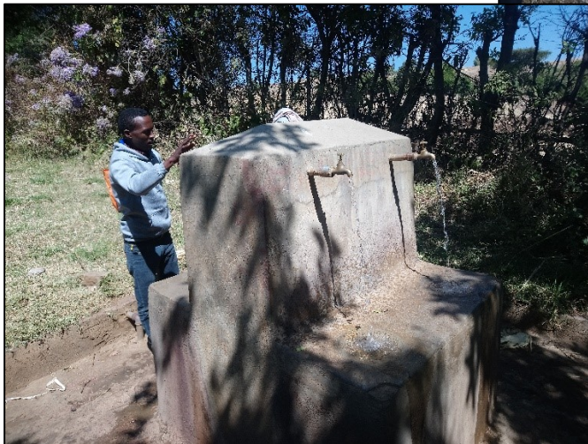
Water collection point with 4 taps. (Photo by Arto, Jan 2019)
