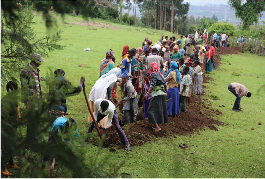
Figure 5.2 Community members provide their labour to dig a trench for their new water supply.
