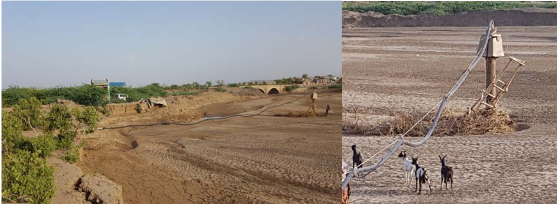
Figure 3-5 Dismantled and eroded well head, pump house... of well located adjacent to Logia river
