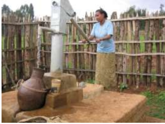
Hand dug wells with hand pump
