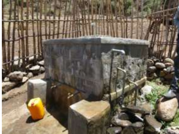
Spring protections with collection chamber and small gravity distribution network with cattle troughs and shower houses
