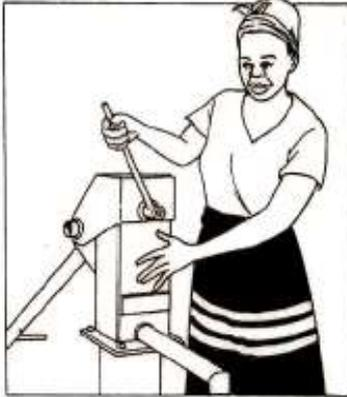
2. Loosen the pump head cover bolt
