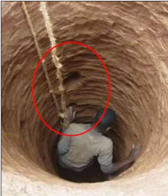
excavation of about 1.5 meters in diameter provides adequate working space for the diggers and will allow a final internal diameter of about 1.2 meters after the well has been lined.
