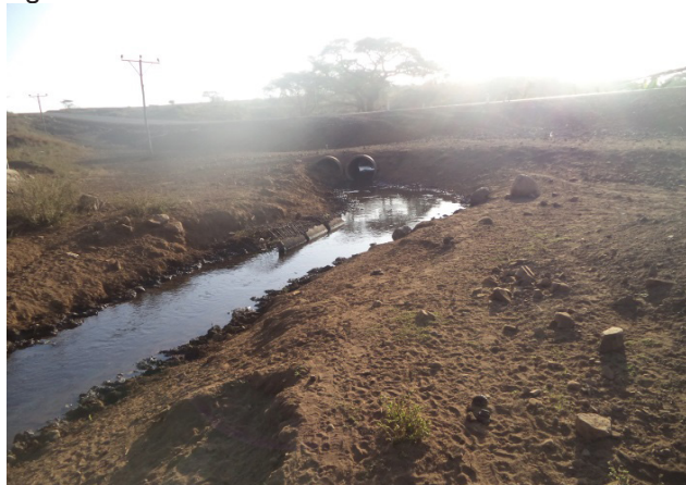
Figure 7. Earthen canal at Hare diversion scheme with no flow control structures.
