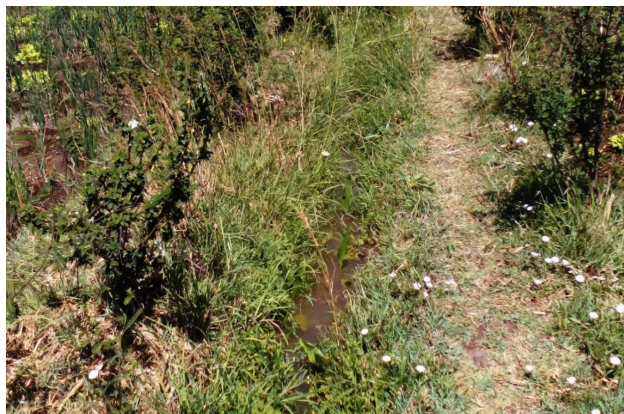
Figure 7. Earthen canal at Hare diversion scheme with no flow control structures.
