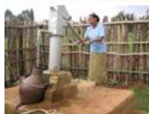
Hand dug wells with hand pump
