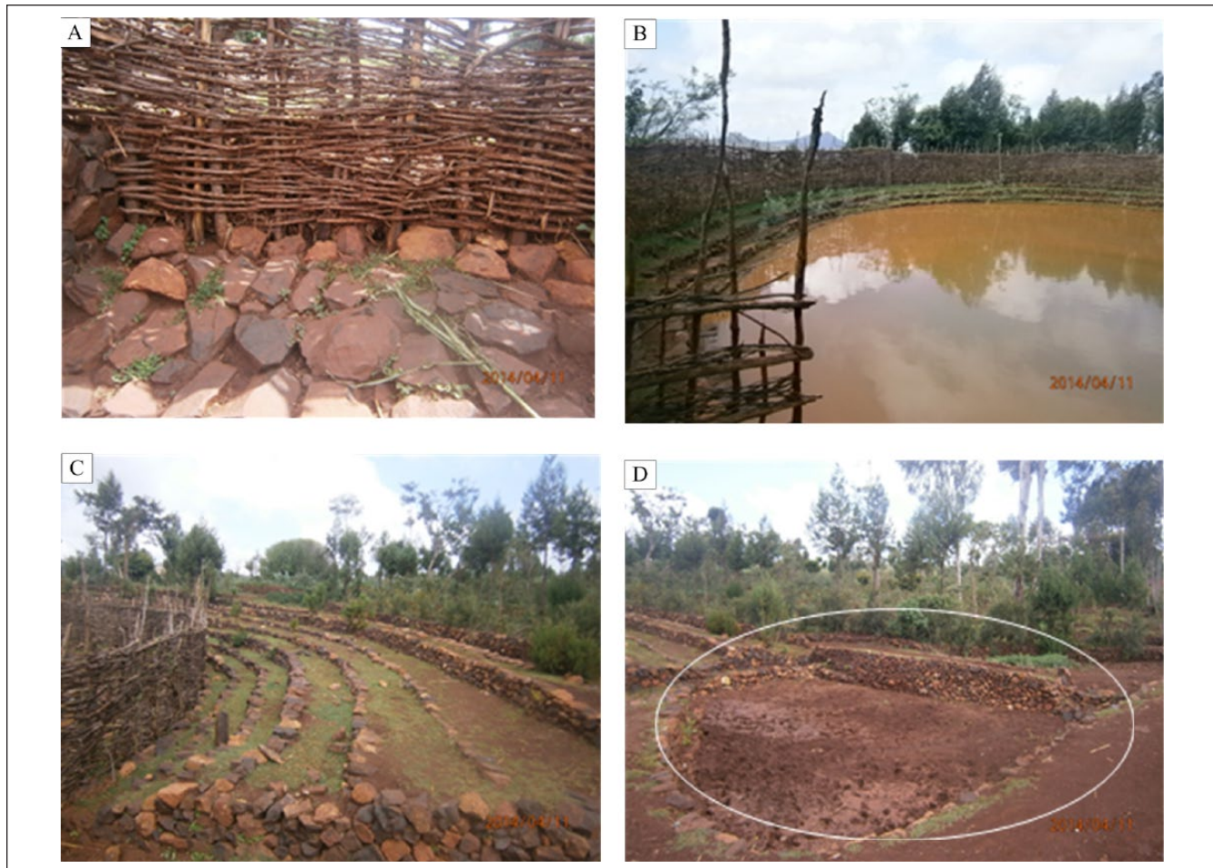
Figure 4. (A) Wooden mesh to filter debris coming to the pond, (B) fenced pond, (C) outside terracing to protect silt from side of the pond, and (D) stilling basin that settles silt coming in with flood before entering the pond.
