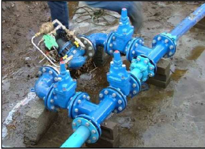
Figure 8: Illustrates typical installation of PRV
