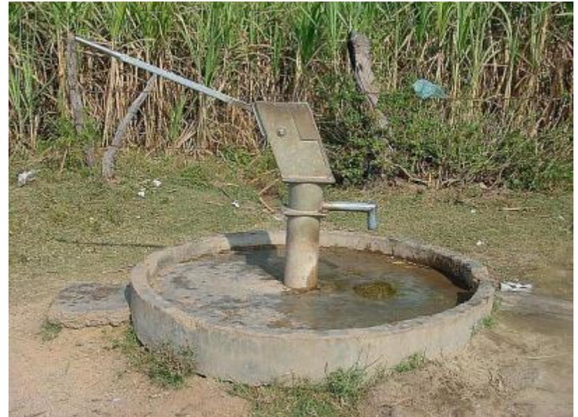
Check with WASHCO if water can infiltrate through the pump or apron which for rope pumps is more easy
