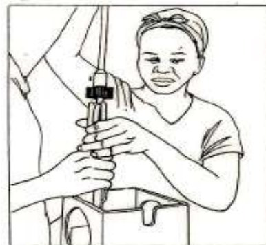
12. Slide the rubber centralizer where the rods join.
