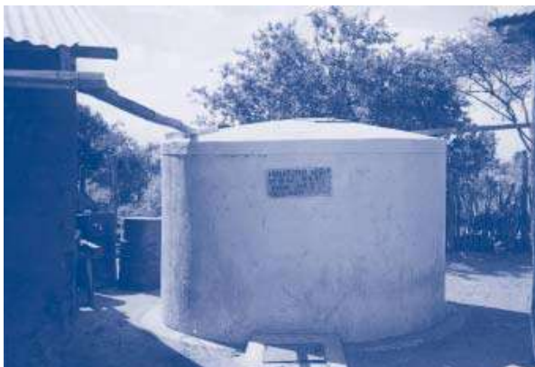
Figure 1.21 Simple roof catchment and storage. Source: IRC.
