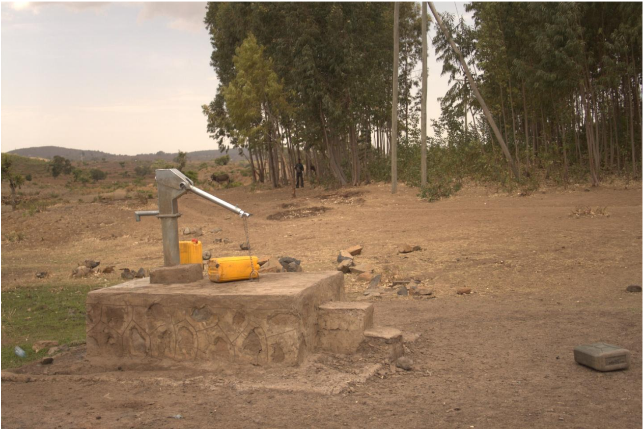
Figure 8: Due to shortage of water abandoned water scheme
